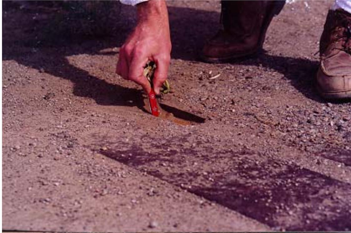
This debris can effect the boundary conditions of the structure and its response to environmental changes
